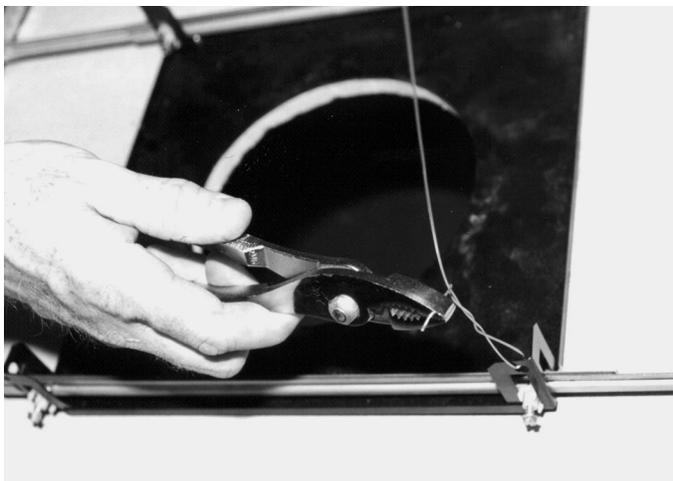
Figure 9.33: Secure Bracket Assembly
