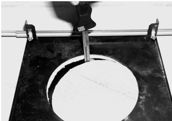
**Figure 9.31: Cut Hole in Ceiling Tile**
