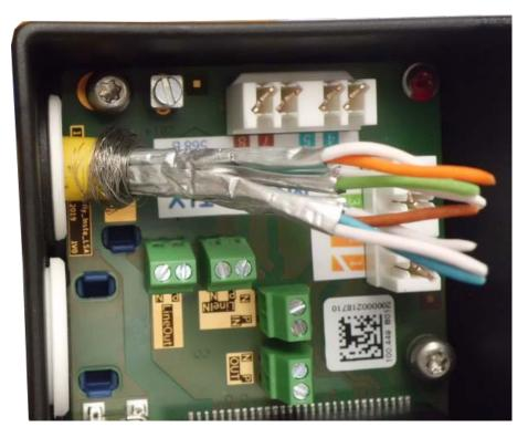
Fig. 60: Network cable inserted, plug properly seated
