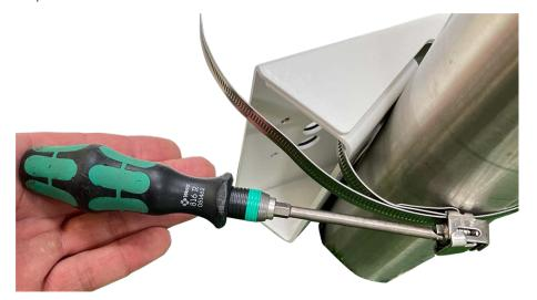
Fig. 42: Tighten the straps
