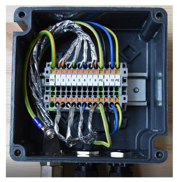
Fig. 5-5 Photo of the occupied terminal box ExTB-3
