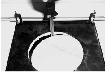
Figure 8.2: Cut Hole in Ceiling Tile
